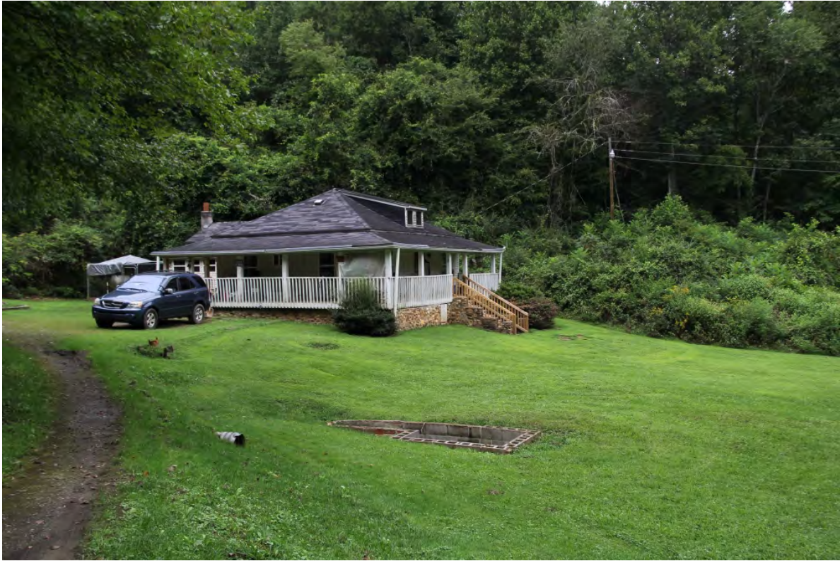
Burnette House, overall view to northwest
