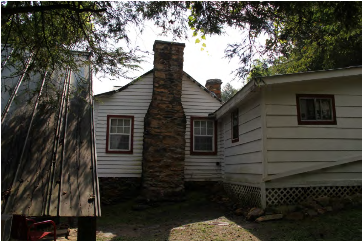
Cobb House, west elevation, view to east
