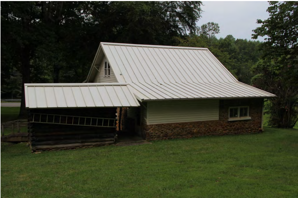
Hatchett House, rear elevation, view to west
