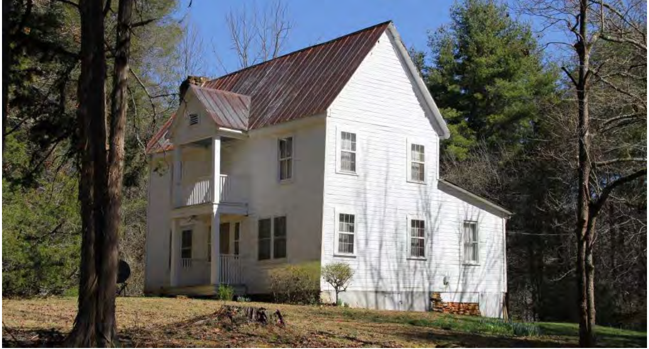
Price-Martin House (CE 165), 697 Lance Road, ca. 1885, oblique view to northeast
