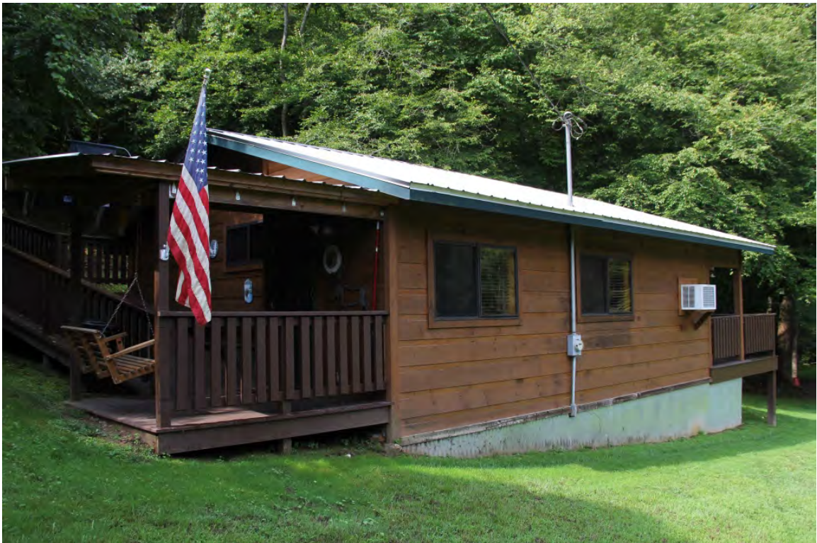
Moose Cabin, ca. 2010, oblique view to southwest
