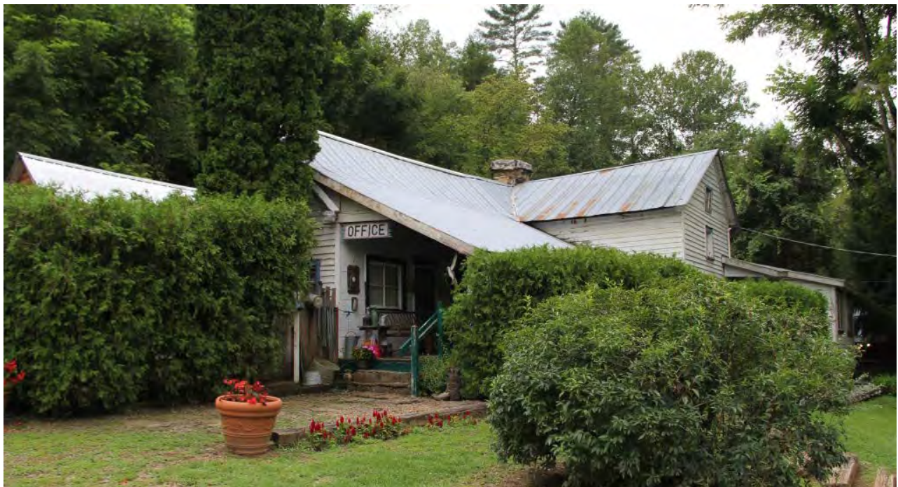
John Franklin Cobb House (CE 33), 106 Cobb Circle, oblique front view to southwest
