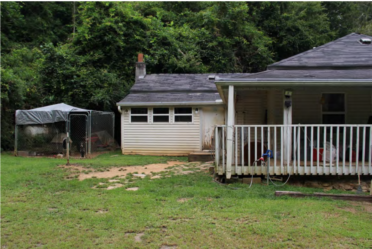
Burnette House, rear ell, view to north
