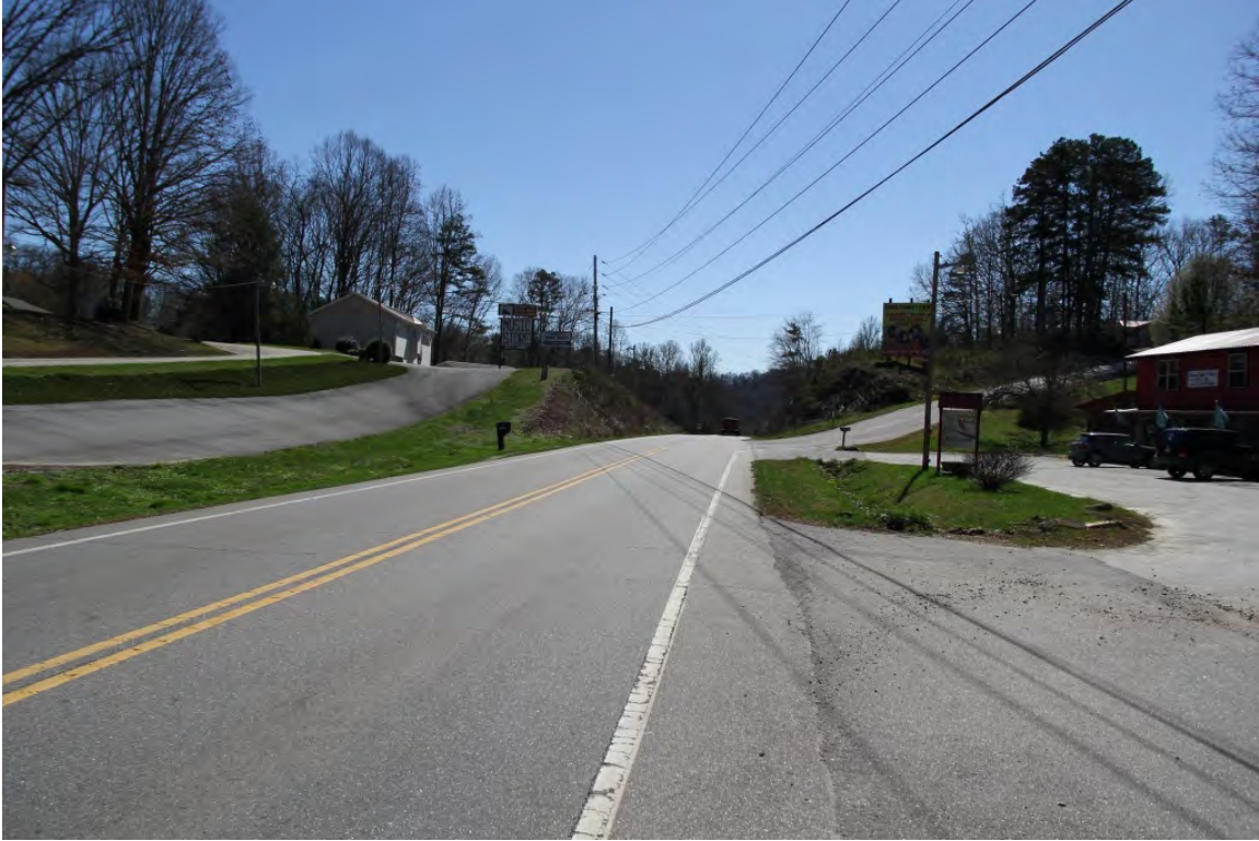
Blairsville Highway (US 19-129) near intersection with Lance Road and Price Weaver Road, view to south
