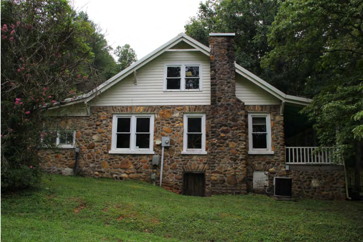
Hatchett House, north side elevation, view to south
