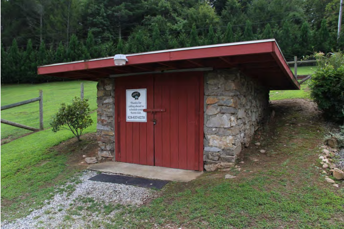
Garage, ca. 1920, façade, view to south
