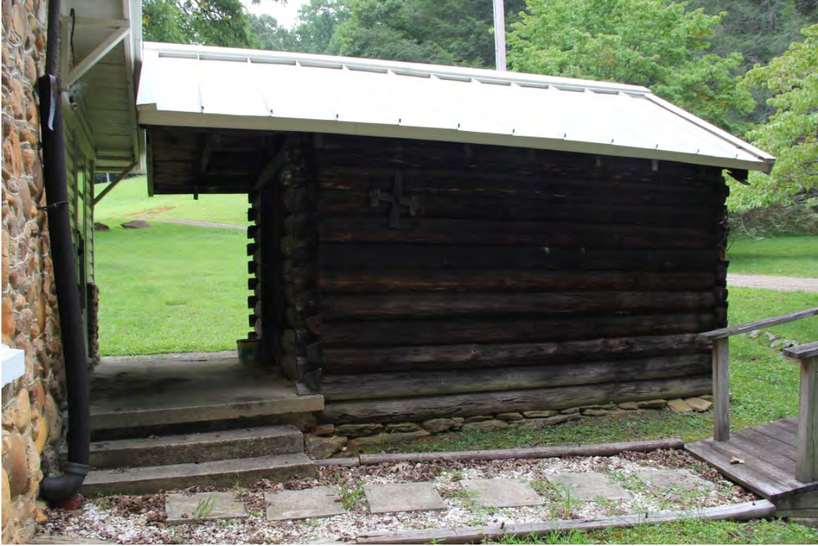
Tool house, view to east
