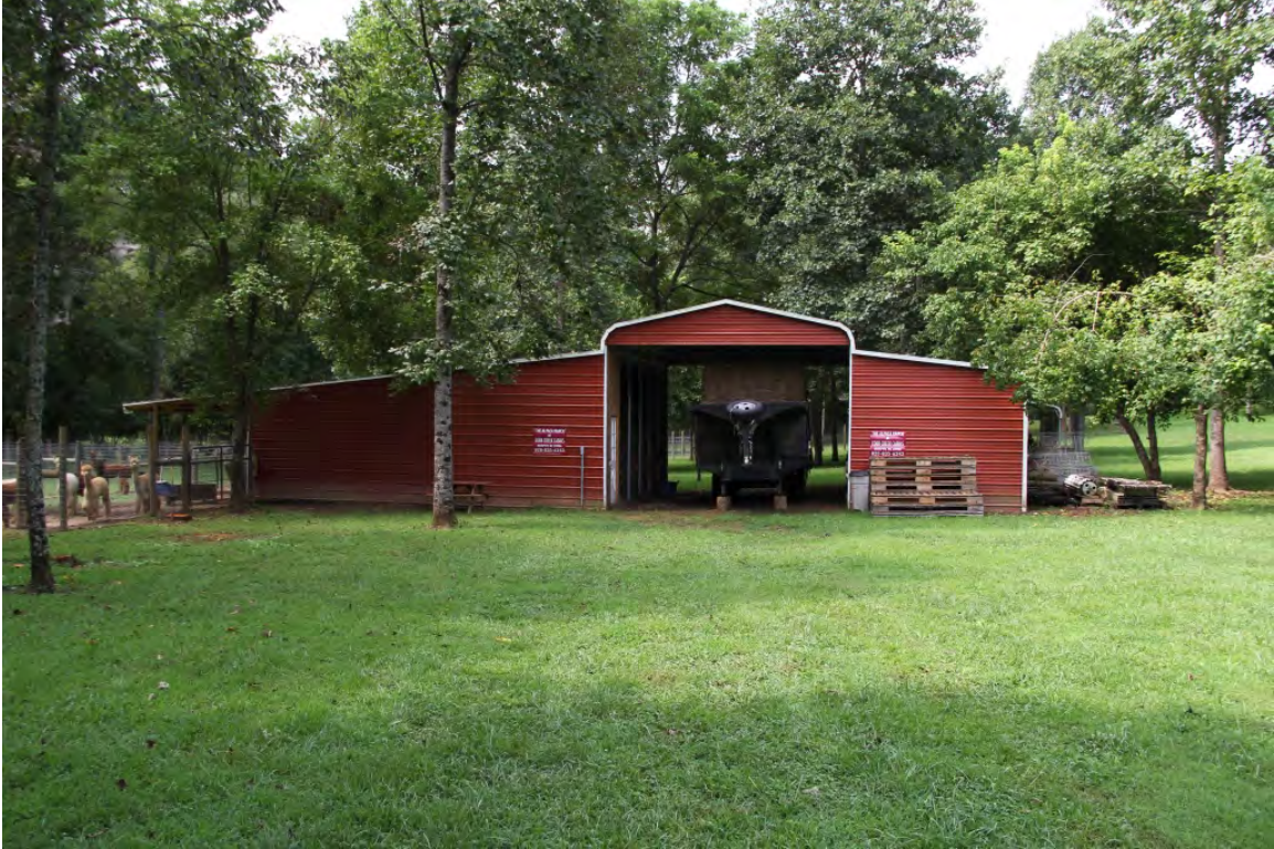
Alpaca Barn (males), 2015, view to southwest
