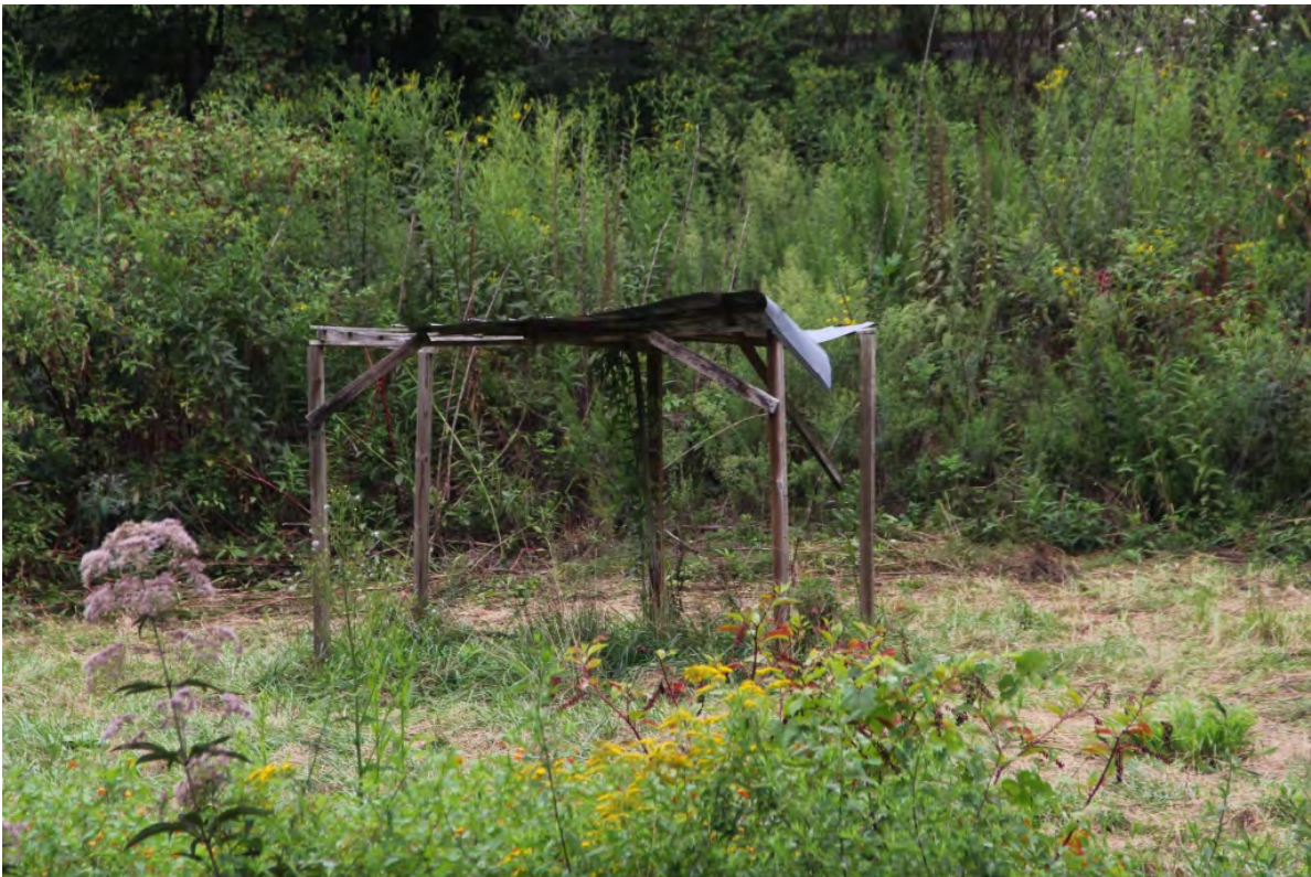
Shed, view to northeast
