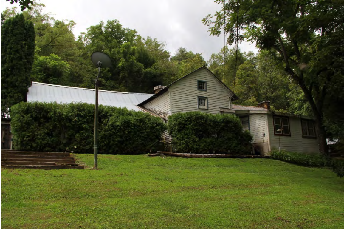
Cobb House, façade, view to southwest
