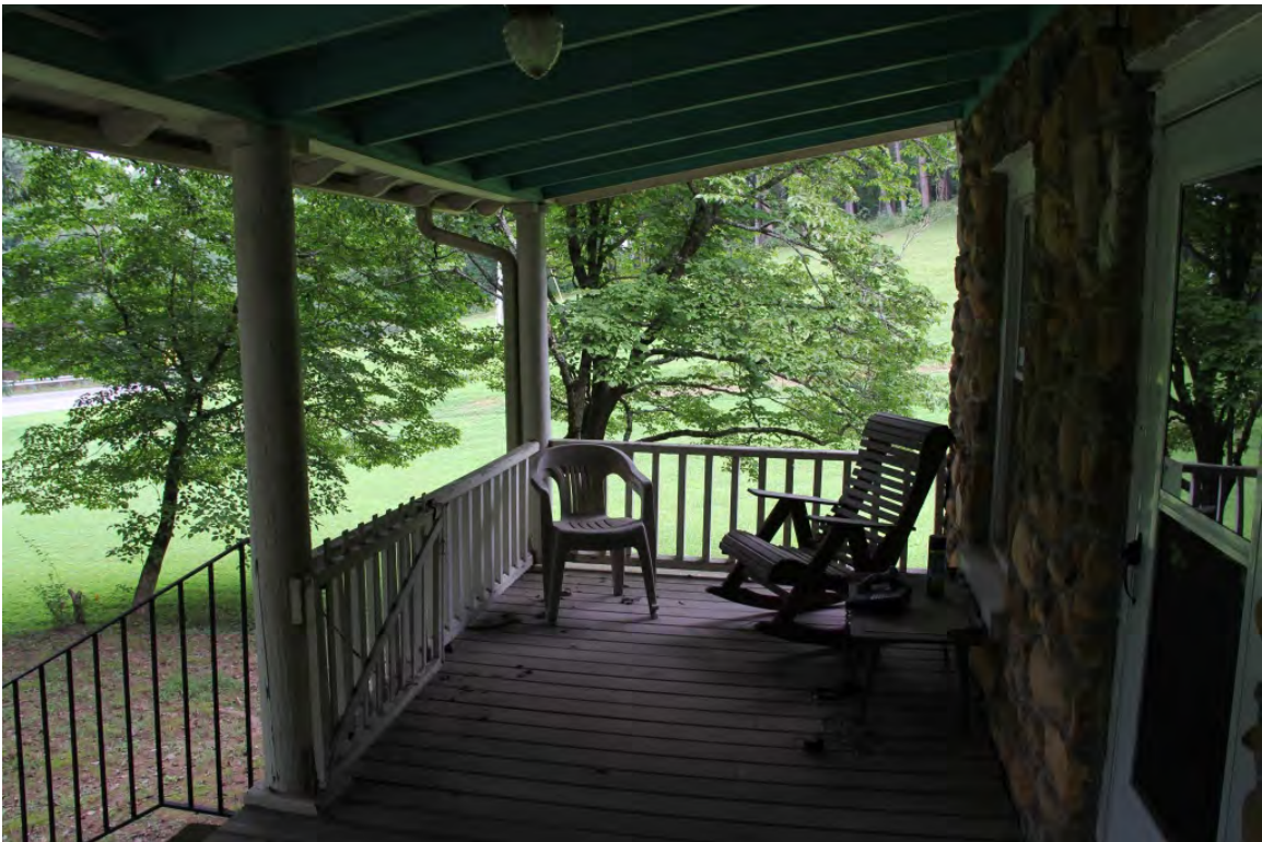
Hatchett House, porch, view to north
