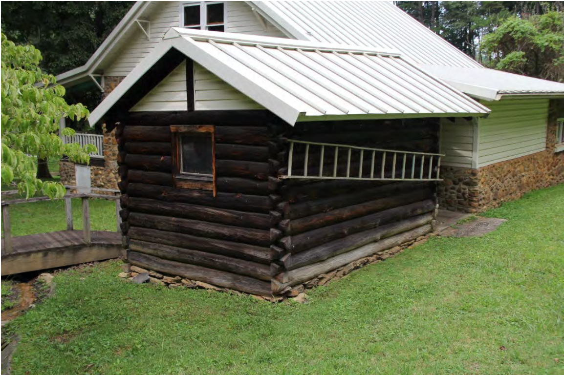
Tool house, oblique rear view to northwest
