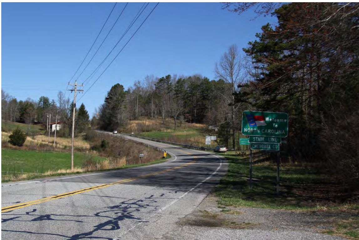
Project beginning, Georgia/NC state line, view northeast along US 19-129 (Blairsville Highway)
