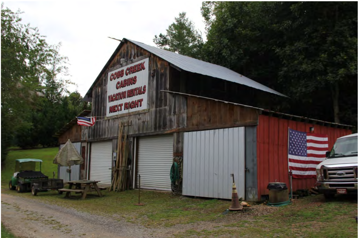
Tractor Barn, ca. 1995, oblique front view to southeast
