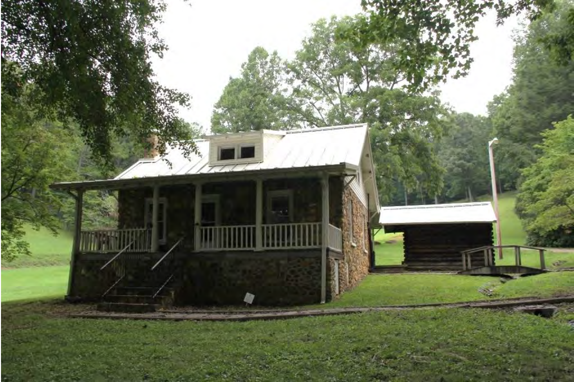
Hatchett House, façade, view to northeast
