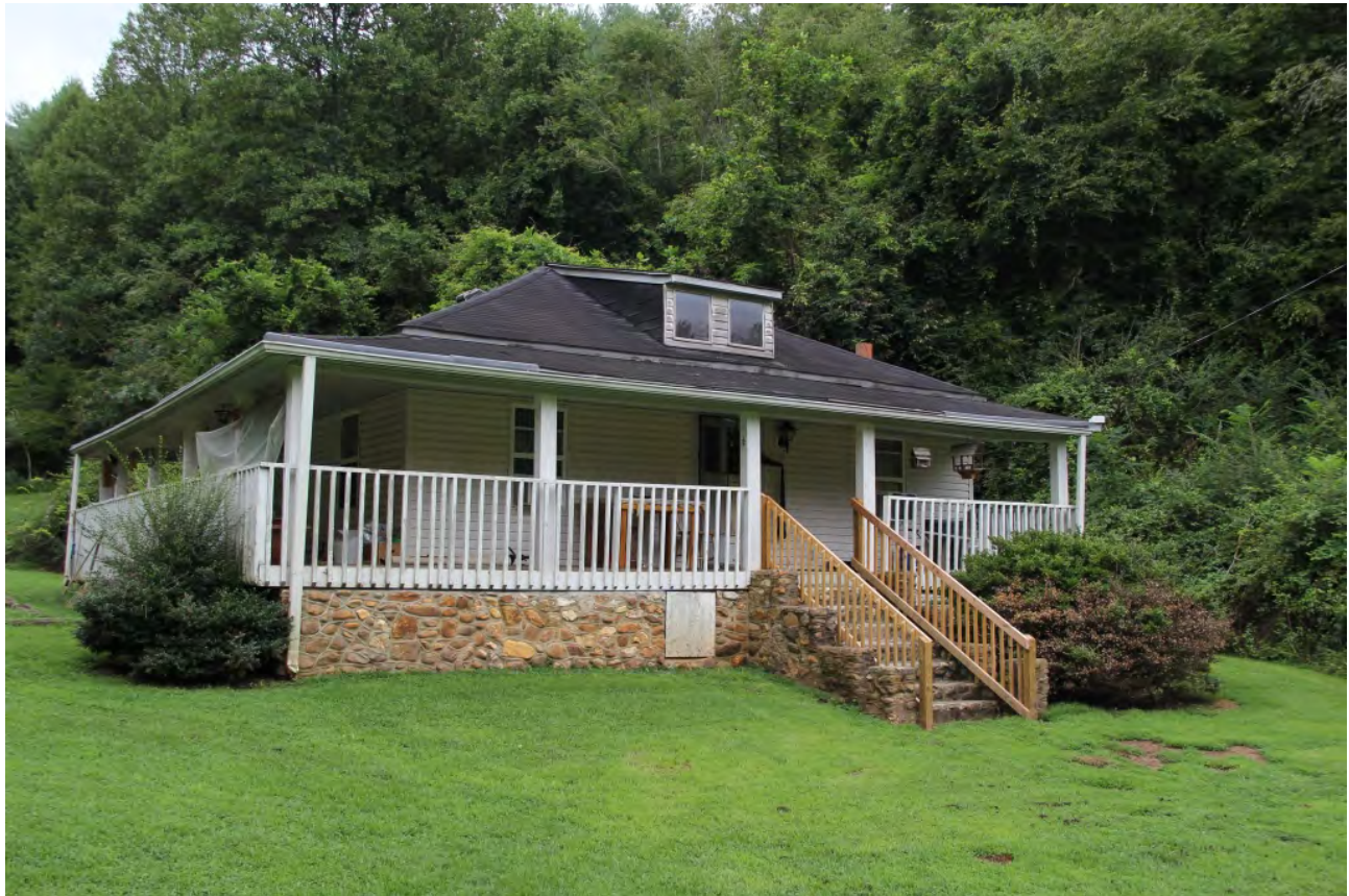
Ernest and Dora Burnette House, 3234 Blairsville Hwy, oblique front view to northwest
