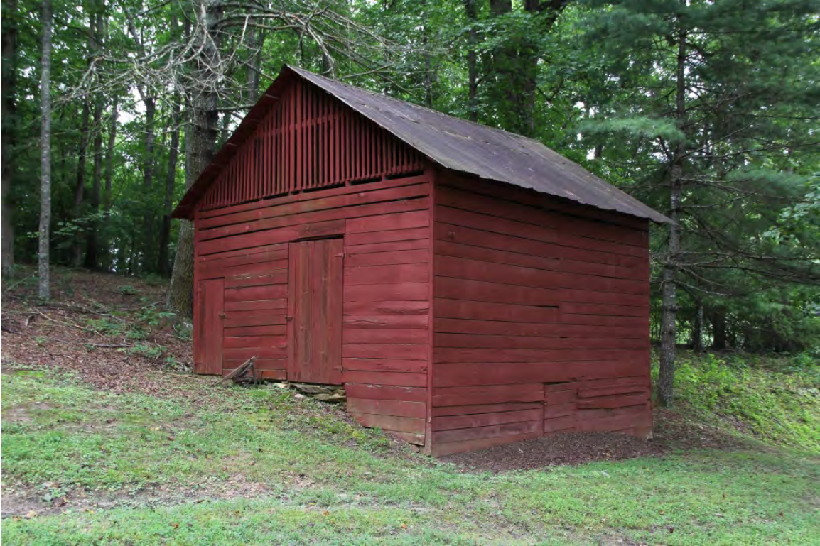
Crib, oblique view to southwest
