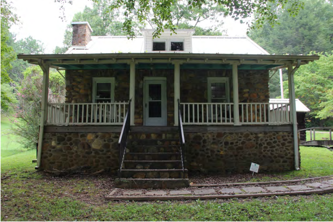
Hatchett House, façade, view to northeast
